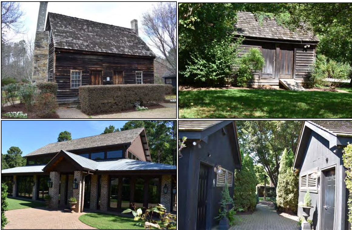
Figure 111: Clockwise from upper left—early house behind main house; early kitchen to rear of early house; frame bathroom buildings (2007); and frame event venue building to north of main house (ca.2016)
