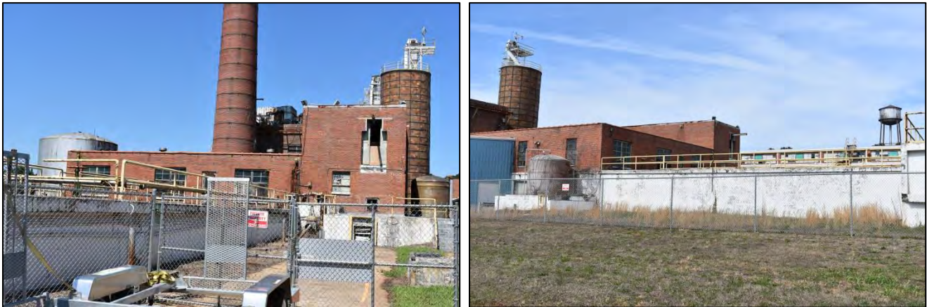
Figure 134: At left, east elevation of pump house, with metal Horton Tank at far left; at right, east and south elevations with concrete wall of water treatment tanks in foreground
