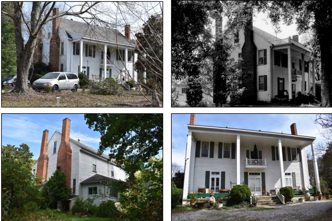
Figure 38: Clockwise from upper left—north side and west front elevations; north and west elevations in 1974; west front elevation; and south side and east rear elevations
