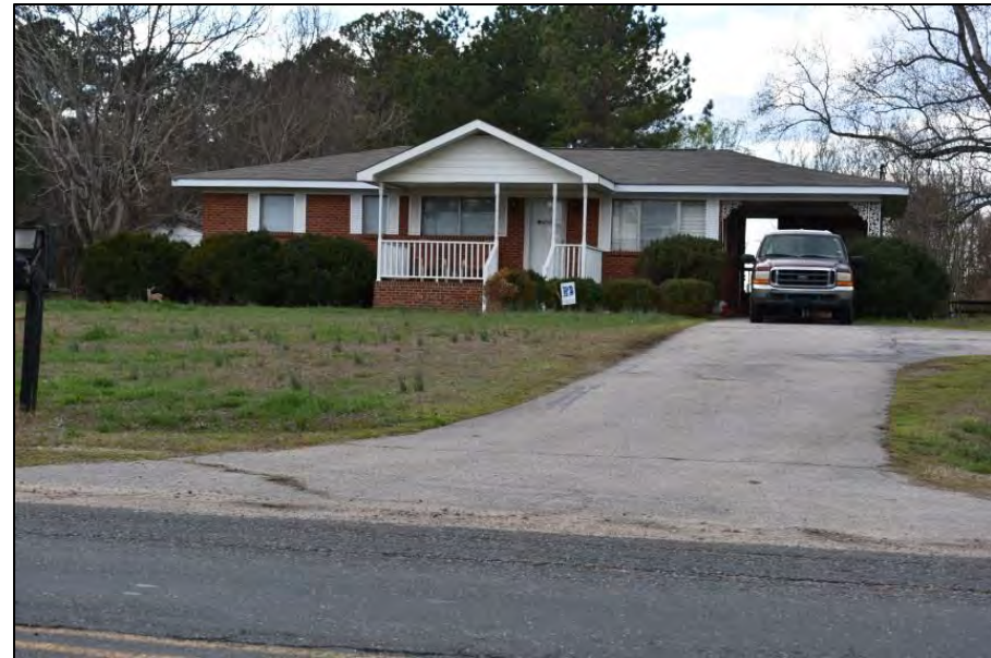
Survey Number: 077 SSN: none Address: 10813 Ponderosa Service Rd. Date: 1953
