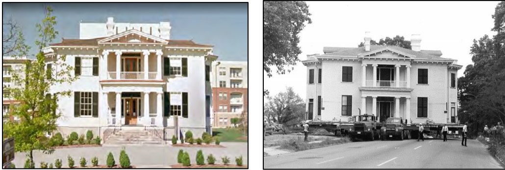
Figure 37: Left, Lewis-Smith House (source: googlemaps); right, house being moved to current location ca. 1974 (SHPO)
