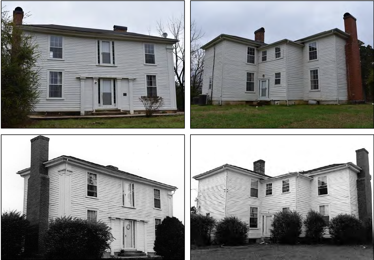
Figure 81: Clockwise from upper left—south front elevation; north rear and west side elevations; north and west elevations in 1988; and front and east side elevations in 1988
