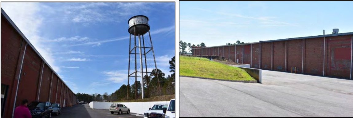
Figure 137: At left, looking southwest at north side wall of original body of plant, with water tower to side; at right, looking southeast at wall toward front of plant, with pilasters highlighted by downspouts
