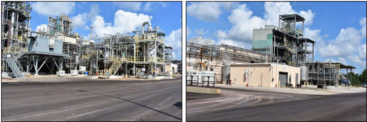
Figure 158: Looking northwest at PAP production plant with, at left, the portion of the facility that contains the ca.1971 building
