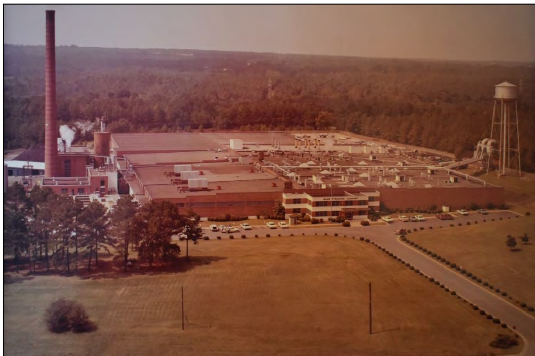
Figure 130: Wake Finishing Plant, ca. mid-1960s; note intact front elevation (Burlington Industries, Inc.)
