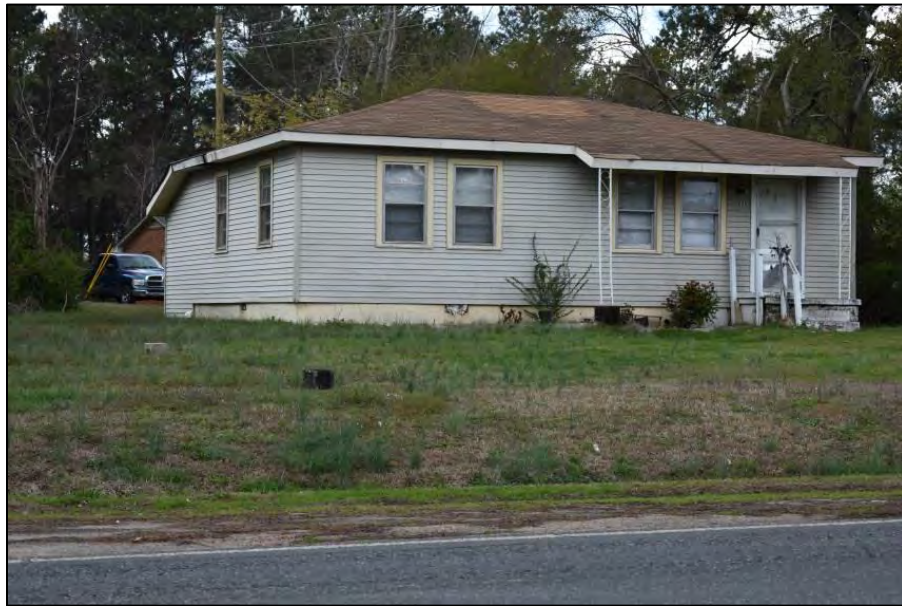
Survey Number: 076 SSN: none Address: 10805 Ponderosa Service Rd. Date: 1959
