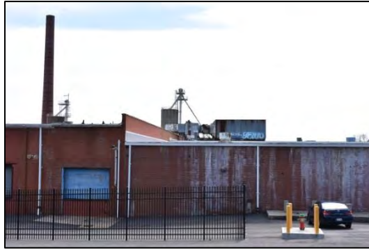
Figure 136: North side walls of 1950s and 1960s additions to rear of facility
