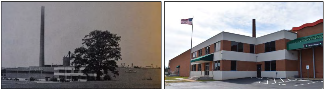
Figure 129: Plant after completion of second expansion, mid-1952 ( Bur-Mil Review , July-August 1952), at left; modern photograph at right
