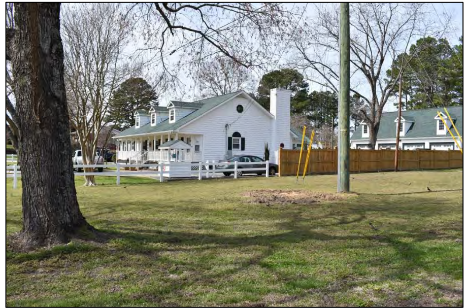
Survey Number: 008 SSN: none Address: 2525 Burlington Mills Road Date: 1960, 1988
