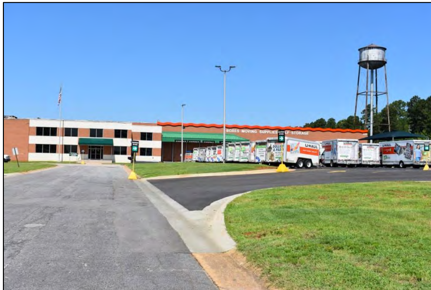
Figure 132: Front elevation with scalloped orange band at eaves added 2017
