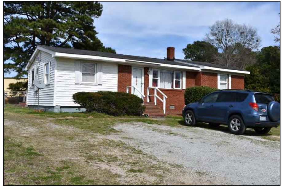
Survey Number: 010 SSN: none Address: 2517 Burlington Mills Road Date: 1960
