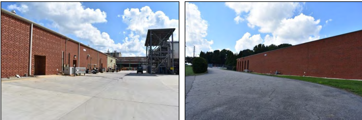
Figure 161: At left, maintenance/workshop building; at right, former pharmaceutical plant building, now used as administration and warehouse building
