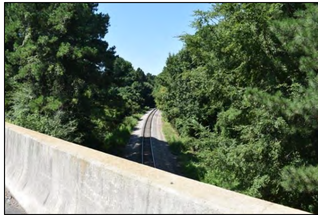
Figure I67: Raleigh & Gaston Rail Corridor looking southwest from US 1 bridge within APE
