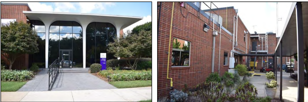
Figure 156: East front elevation of office building, at left, and west rear elevation, at right
