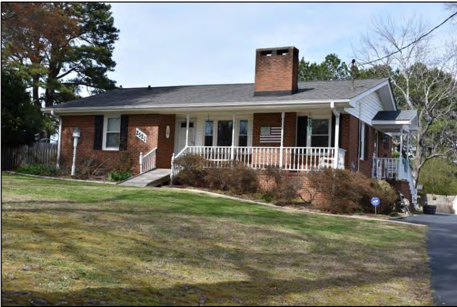
Survey Number: 009 SSN: none Address: 2521 Burlington Mills Road Date: 1963
