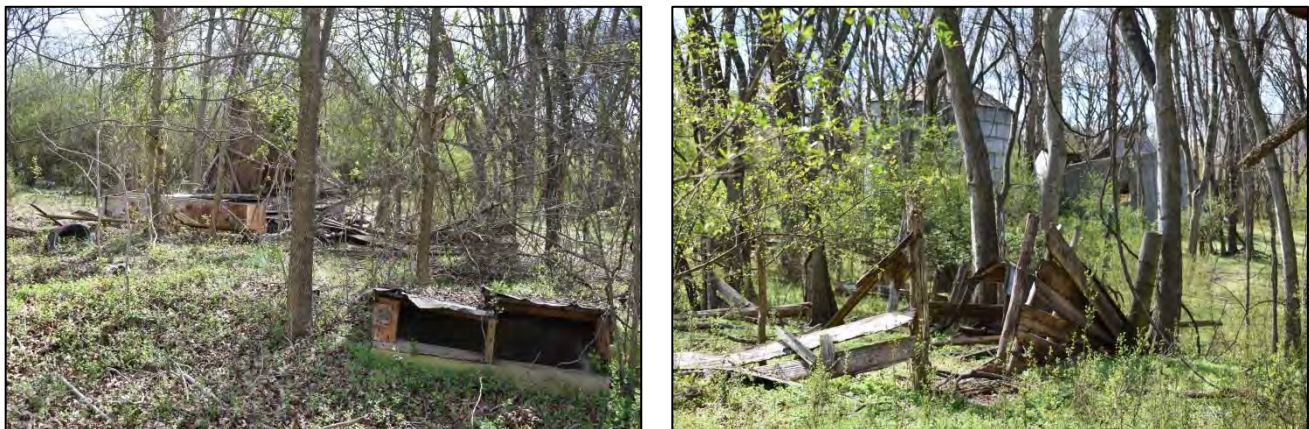
Figure 26: Ruins of early/mid-twentieth century farm buildings
