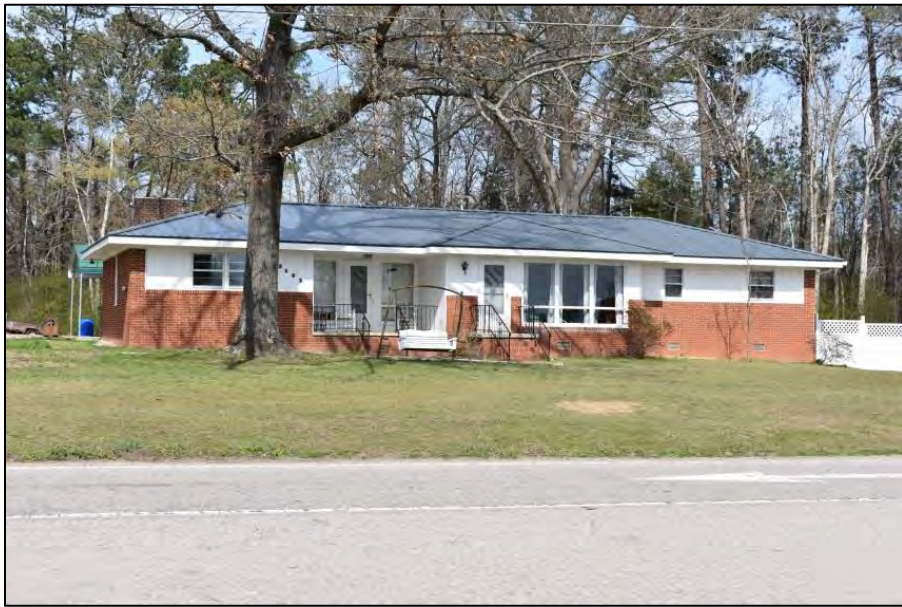
Survey Number: 007 SSN: none Address: 2605 Burlington Mills Road Date: 1963
