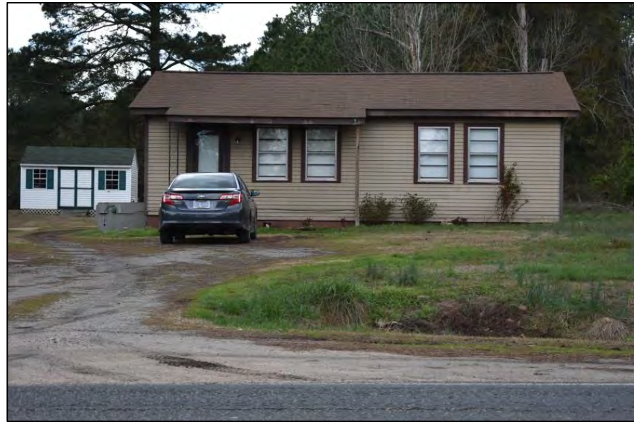
Survey Number: 075 SSN: none Address: 10801 Ponderosa Service Rd. Date: 1959
