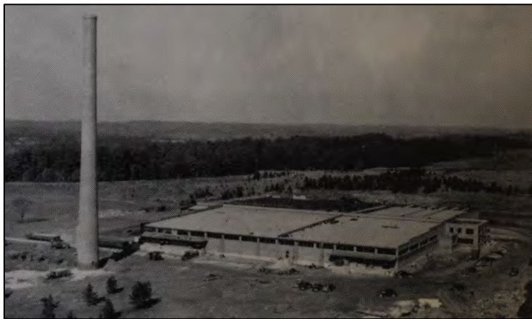
Figure 143: Wake Finishing Plant under construction, early 1948 ( Bur-Mil Review , February 17, 1948)
